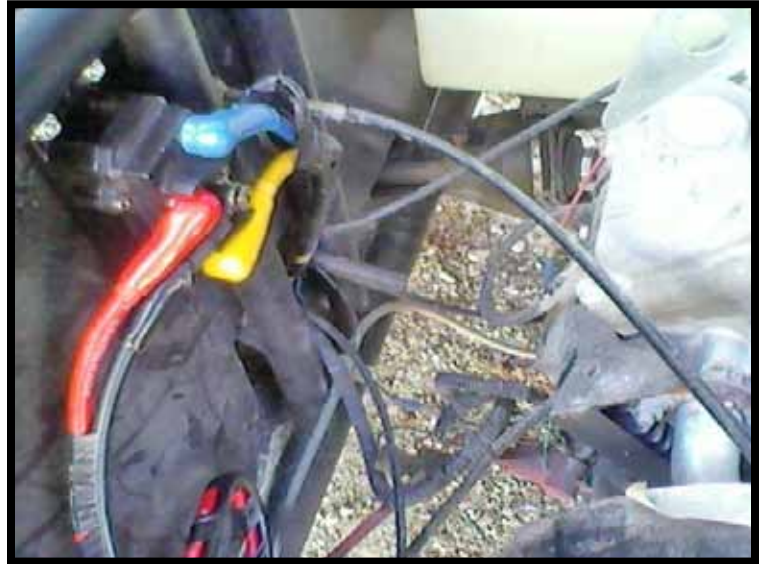
“Figure 7” Contactor Location
